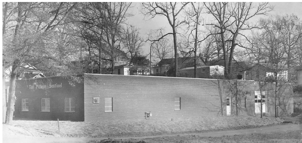
In 1968, this was a new building for The Pickens Sentinel newspaper, at that time owned by the Hiott family. It is now the location for Hiott Printing, on Johnson Street in Pickens.
